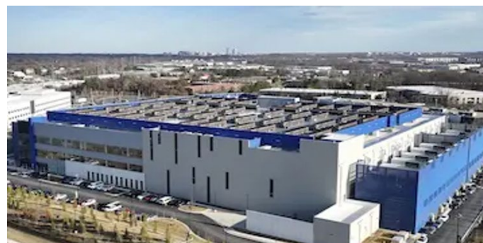
Digital Bridge – Data Center Fund Investment Sterling, VA
