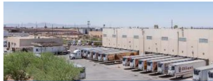
Martin-Brower Cold Storage and Distribution Facility Phoenix, AZ
