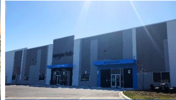
Amazon Last Mile Distribution Facility Cleveland, OH
