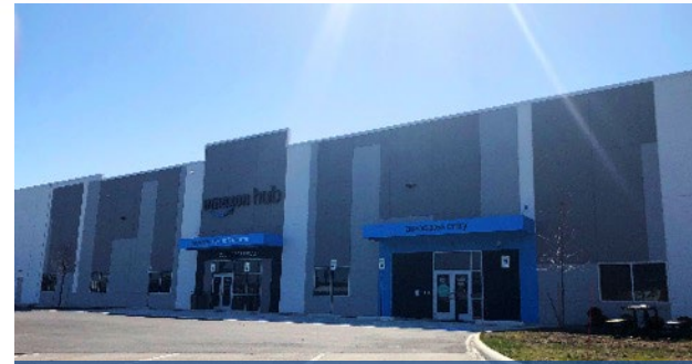
Amazon Last Mile Distribution Facility Cleveland, OH
